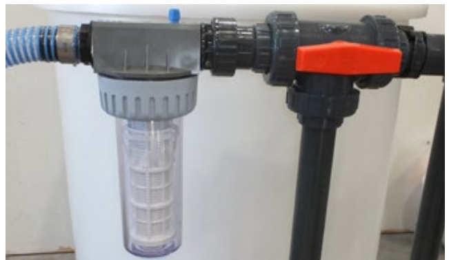
Heavy duty filter and 3-way valve
